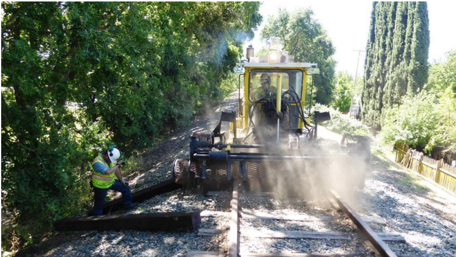
Heather digs out a tie-crib
