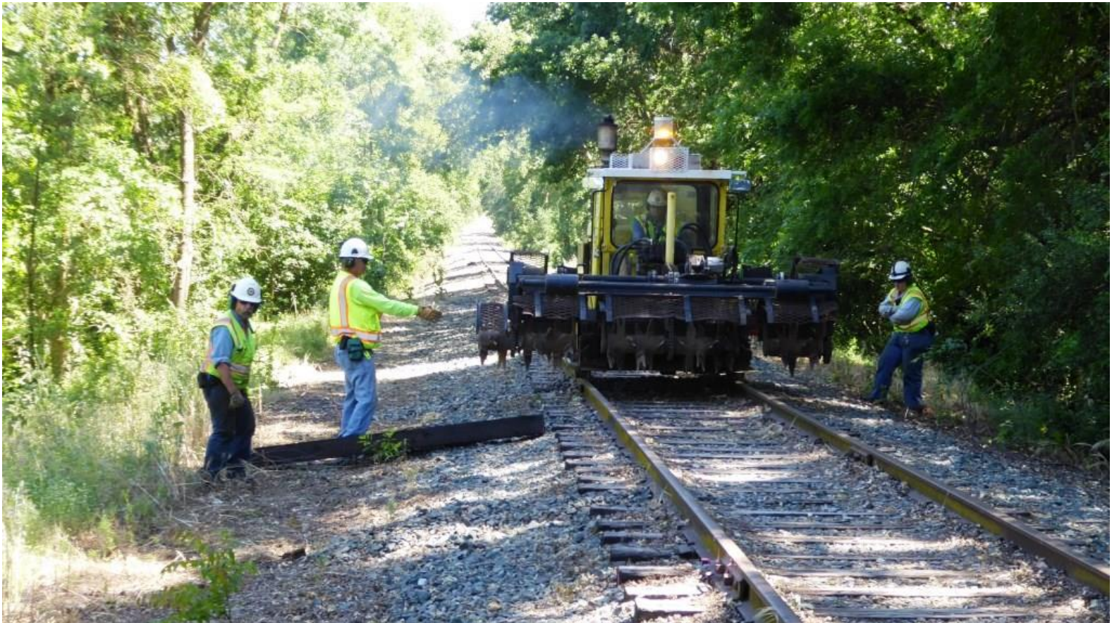
Last tie of the day: Taka guides Kyle in the scarifier to line-up with the empty crib where he and Joe will guide it into position
