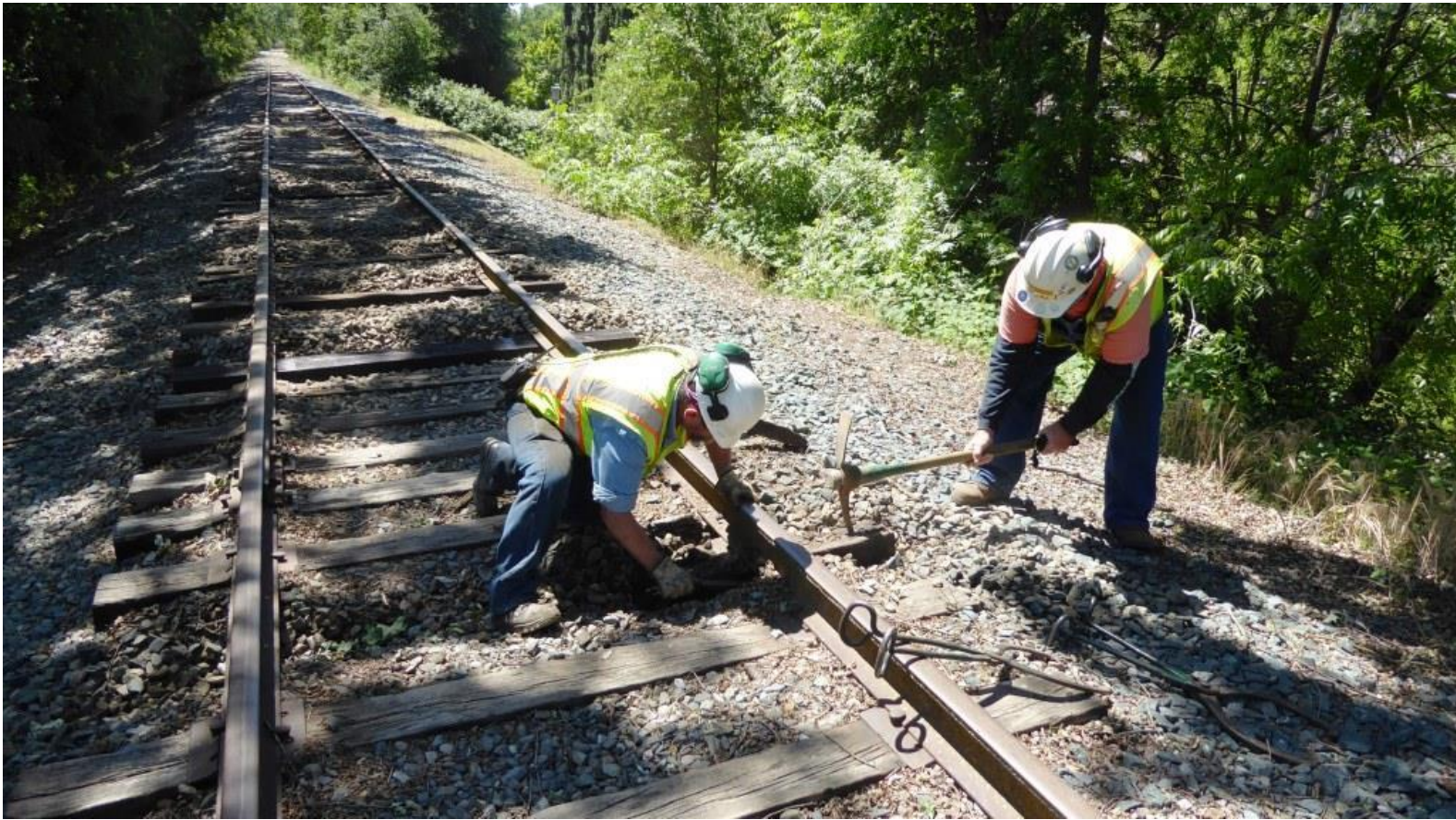
Joe and Mike F. remove the remnants of half a tie that broke in half when being pulled
