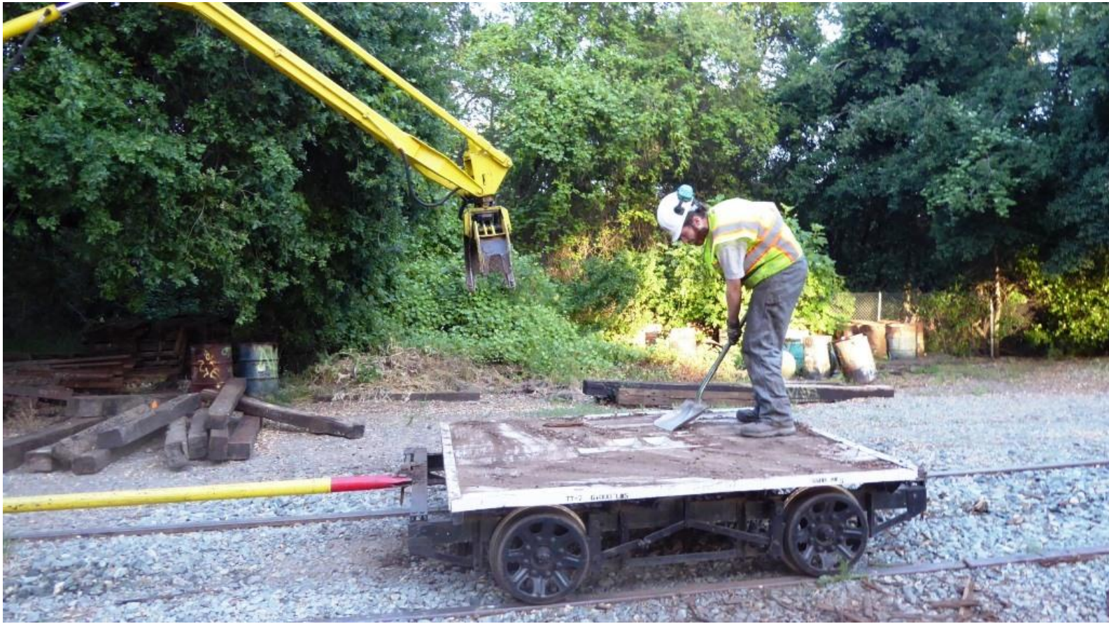
Matt cleans dead-tie debris off of the flatcar
