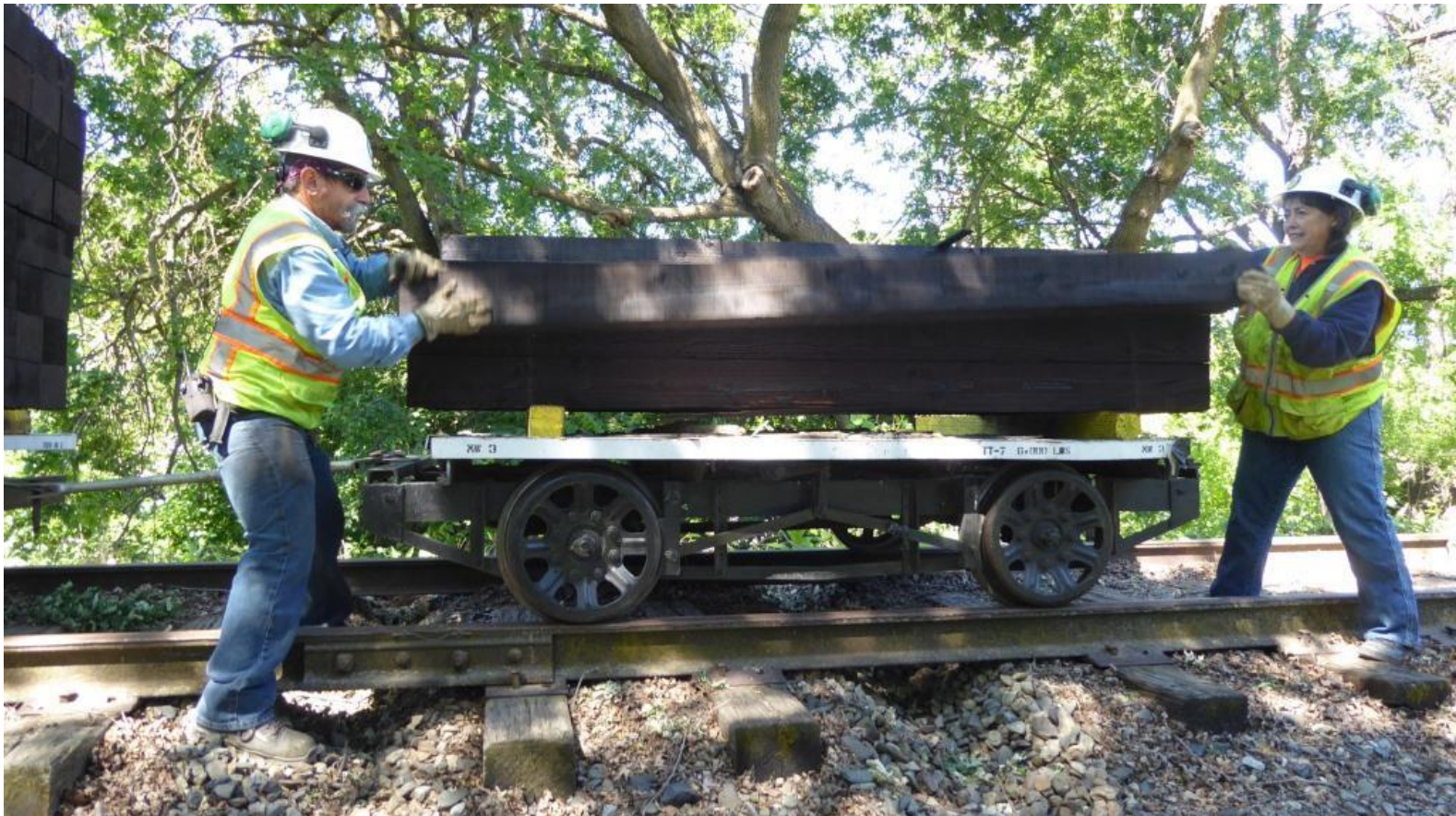
Joe and Pam drop ties off the flatcar and spot them near the empty tie-cribs
