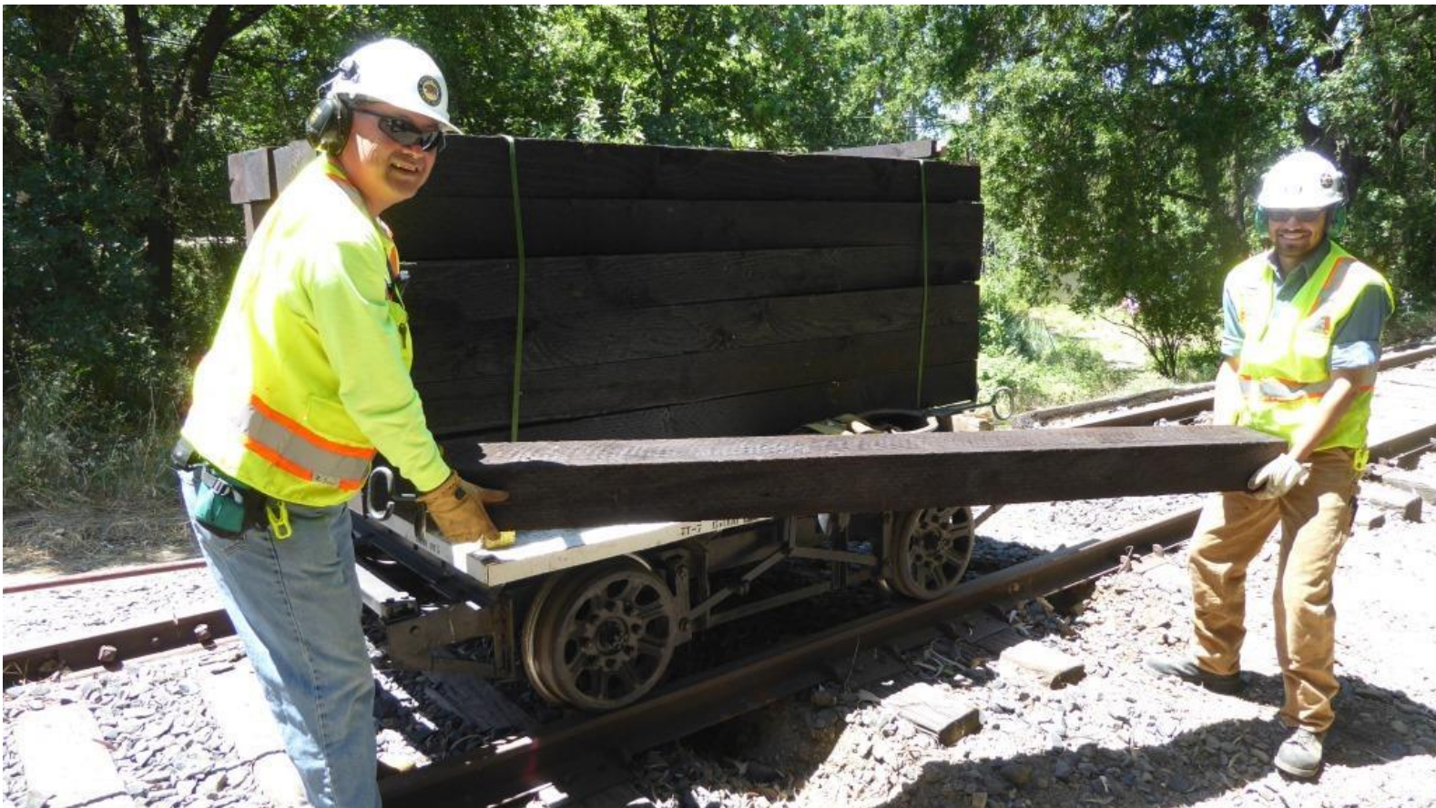
With the discovery of about 20 cribs that we missed, Taka and Kyle move more ties into position for installation
