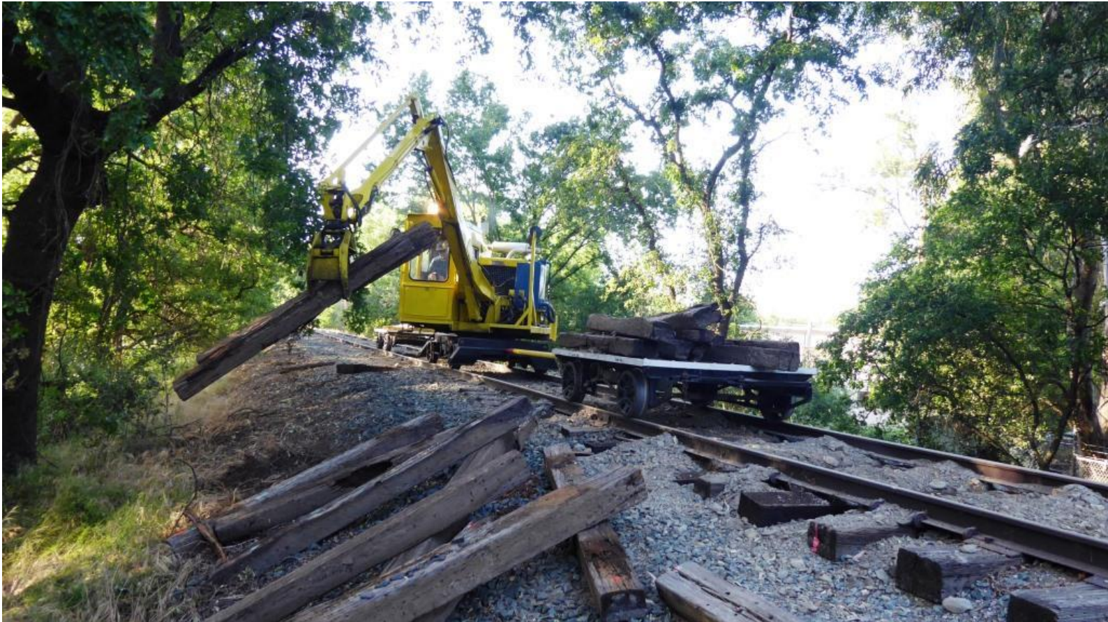
Alan in the Tie-crane removing dead-ties strewn about the Sutterville Line track
