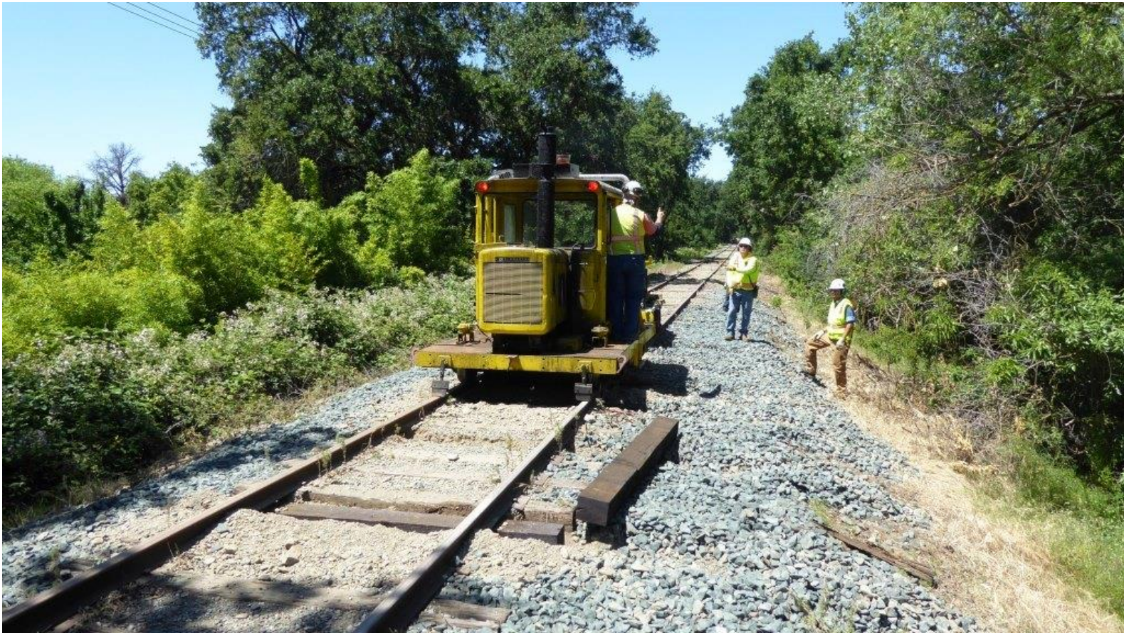
Taka requests a "red-zone" which Engineer Mike F. on the Kalamazoo acknowledges
