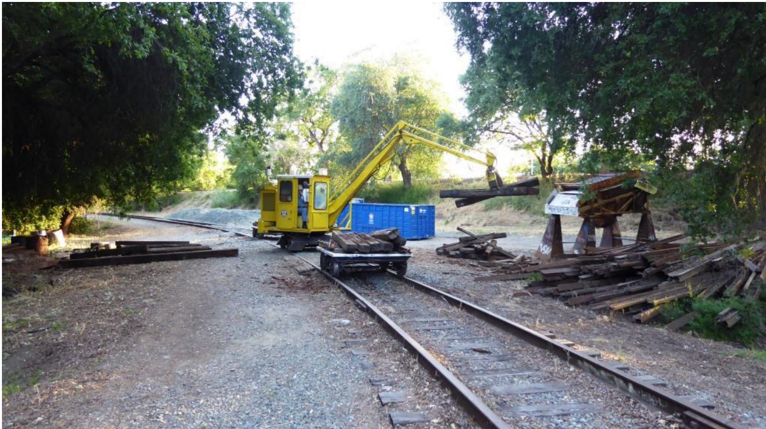
At Setzer, Alan transfers the dead-ties from the flatcar to the new and growing dead-tie pile
