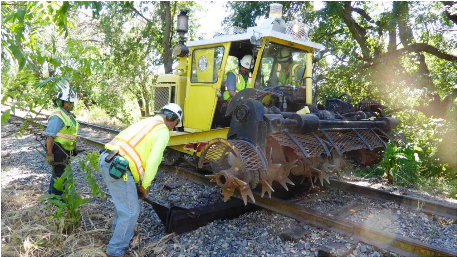
Kyle operates the scarifier-inserter as Taka guides a tie under the rails
