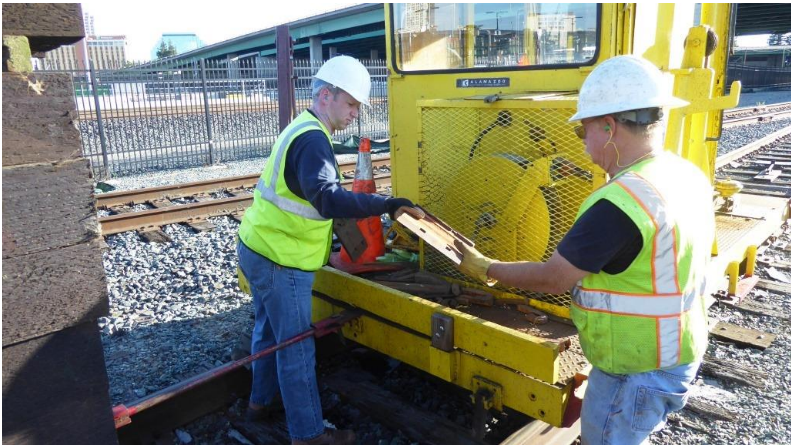
Kevin and Mike H. transfer the pile of tie-plates from the deck of the Kalamazoo into a wire basket
