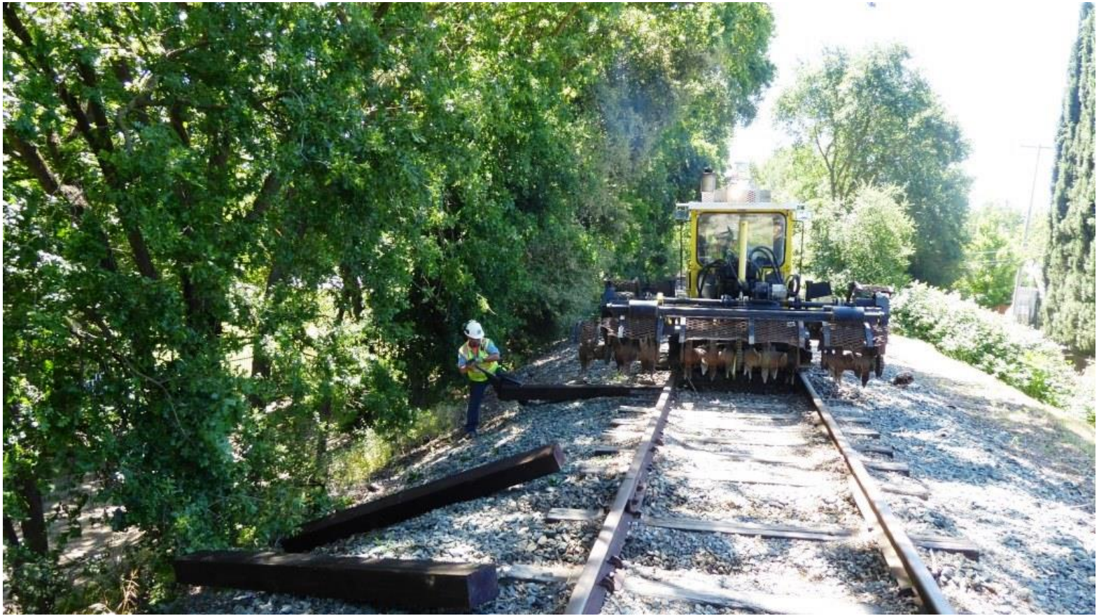
With ties deployed, Joe guides a new tie under the rails which Heather, in the scarifier-inserter, pulls into place
