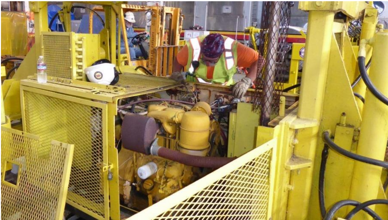
Joe digging into the inner-workings of the Jackson 125 Tie-exchanger
